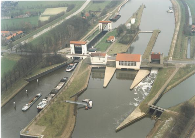
Figure 3. The canal lock (left hand side) and the water pumping station, source: RWS
